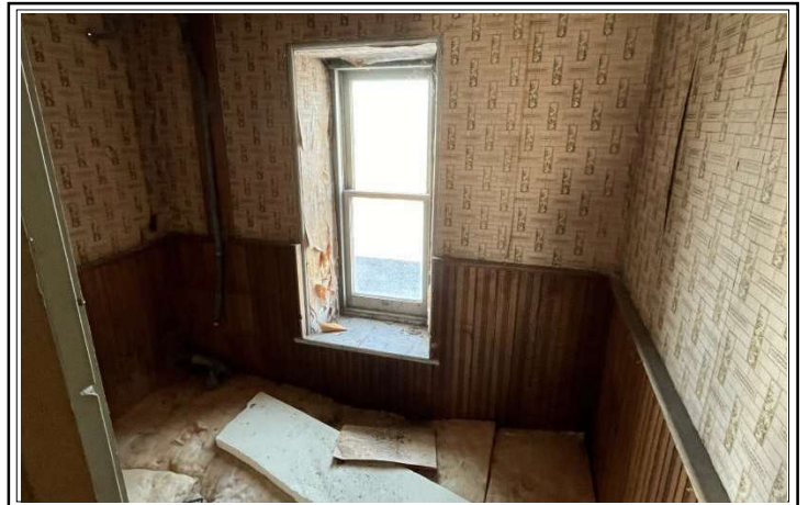
Interior View - Rough-In Washroom
