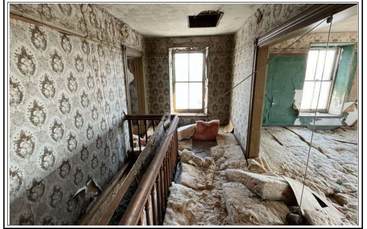
Interior View - Third Level Landing
