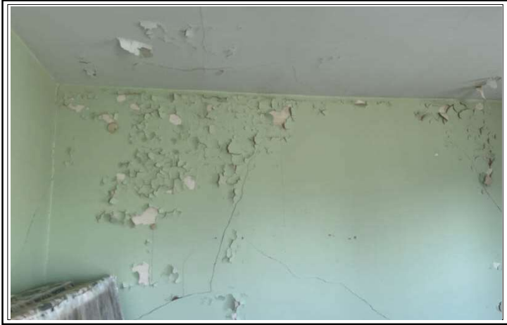
Chipping Plaster / Painted Walls and Ceilings
