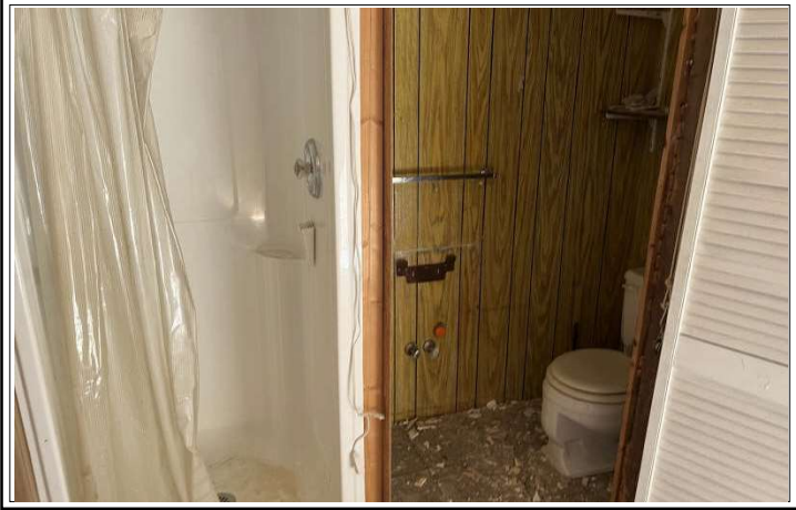
Interior View - Washroom
