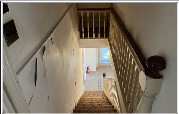
Chipping Plaster Walls
